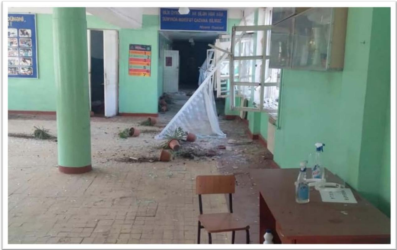
Photo 9: Damaged elementary school in the Ganja city
