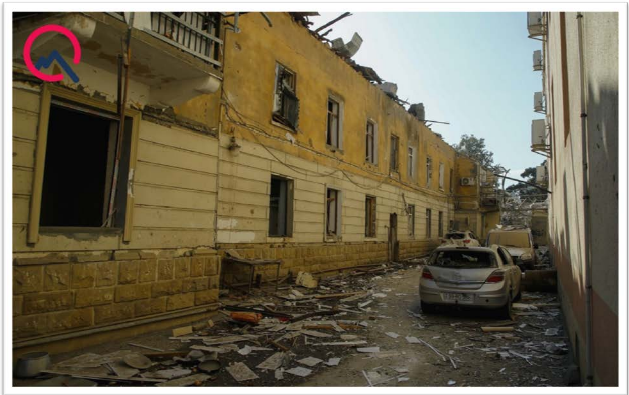
Photo 29: Damage inflicted upon the civilian infrastructure in the city of Ganja
